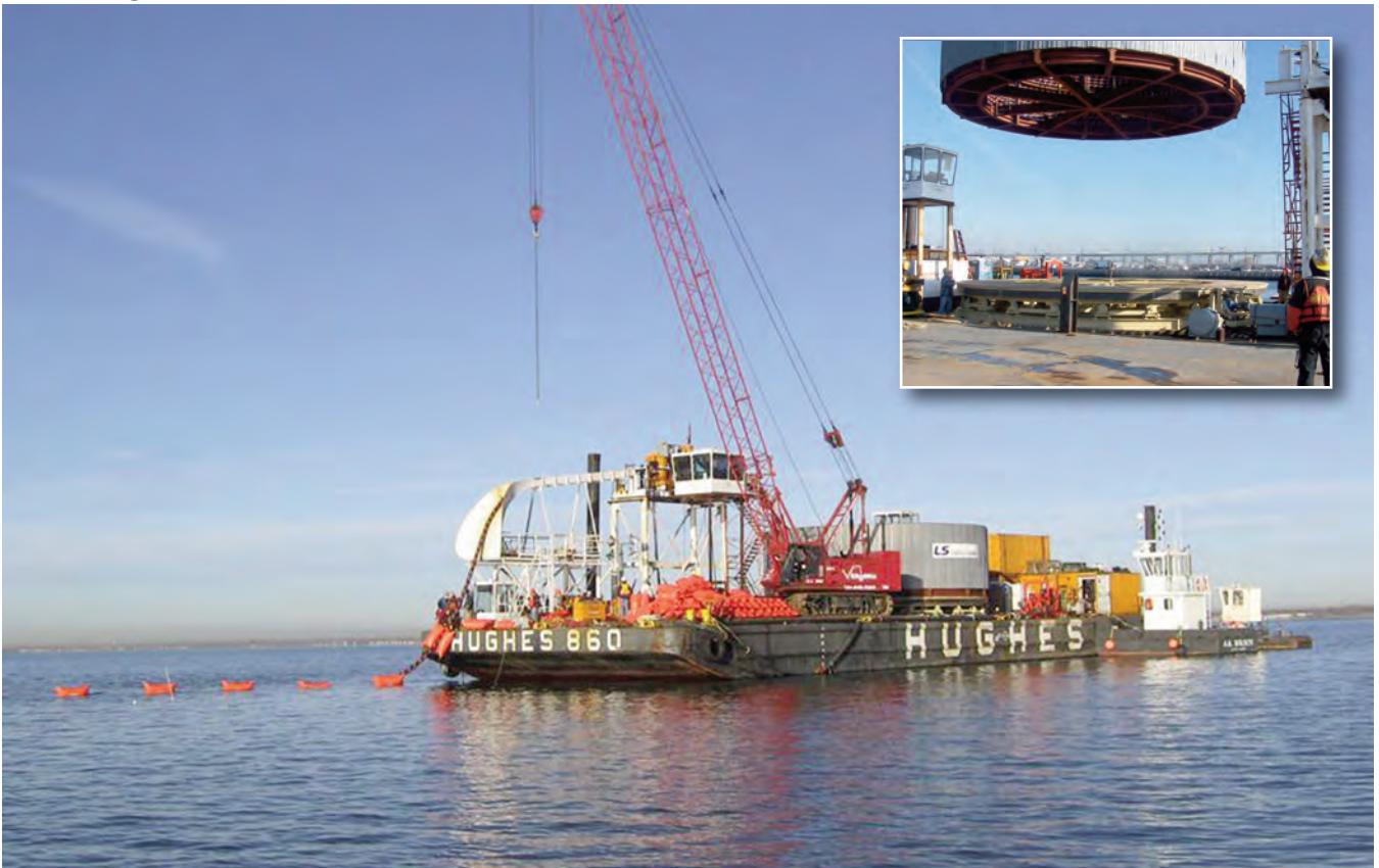
Cable being installed from turntable.
